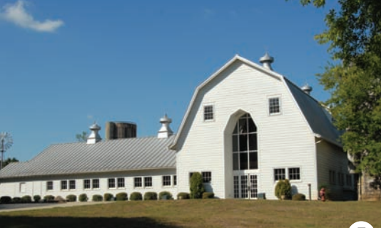
Dairy Barn 35° 2'43.50"N 80° 55'56.00"W
